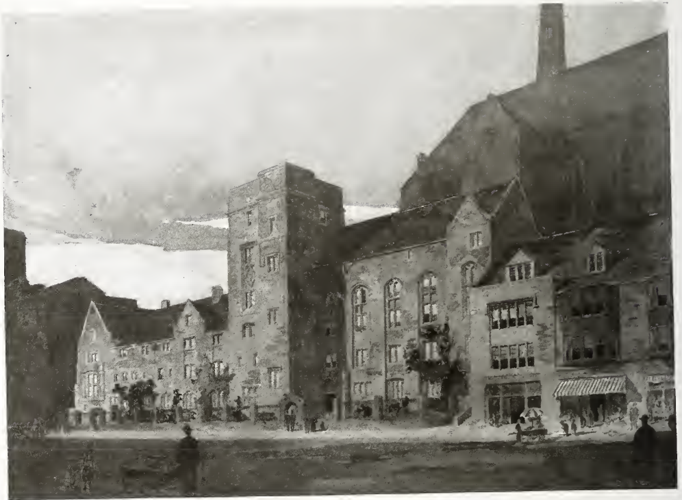
EXTERIOR—THE COMMUNITY HOUSE, ETC., OF THE PAULIST FATHERS, NEW YORK CITY. New York Office, 1907.
